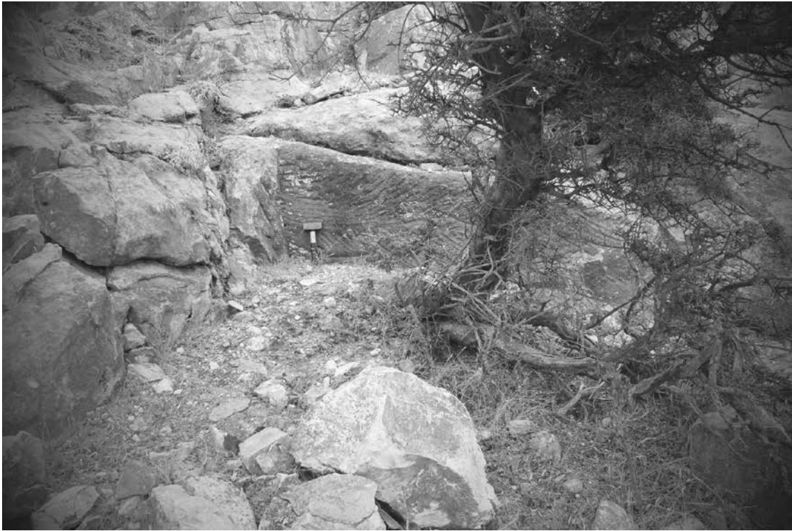
Fig. 8 - Detail of a vertical cut showing marks of the Roman heavy pick
